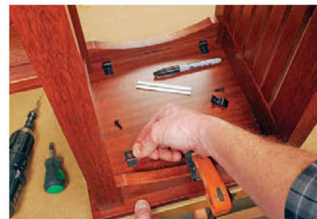
Attach the top panels and shelves to the arched rails with a pair of tabletop fasteners installed in each rail's kerf. Be sure to account for how the panels will need to expand or contract when locating the fasteners.
